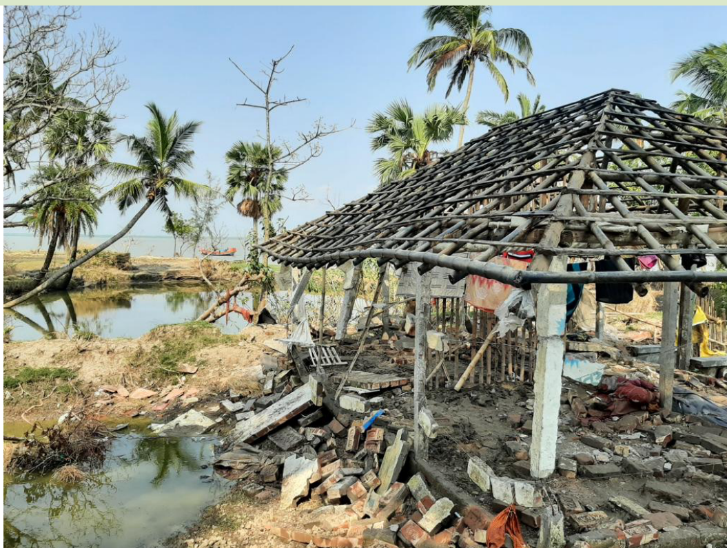
Damaged house and flooded land after Cyclone Yaas. Photo by Pinaki Halder/Landesa, 2021.
