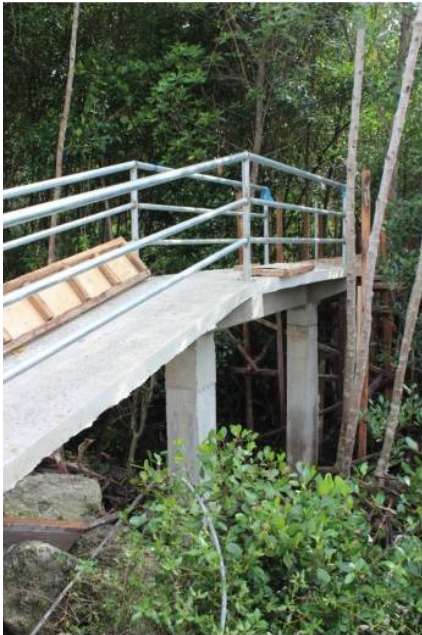
Boardwalk constructed under the CBFMA project photo by IJFR
